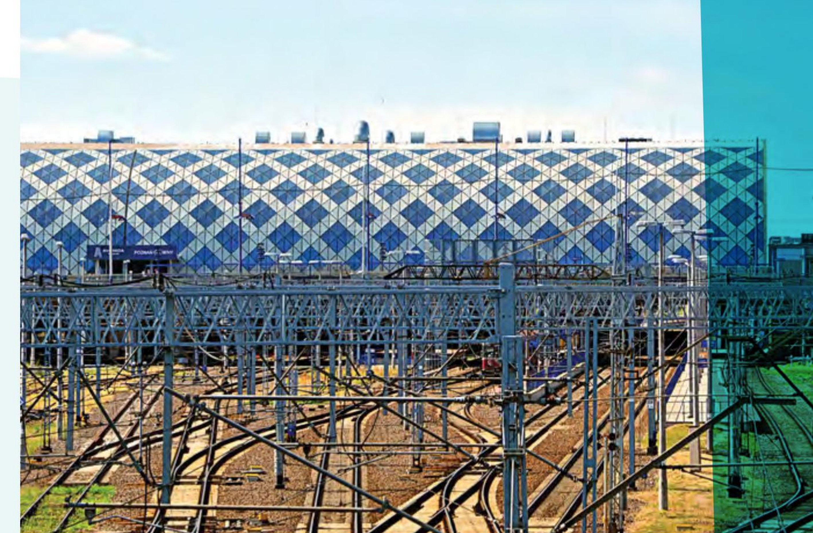
It extends on the somewhat clandestine platform 4B. Just follow platform no.4 northwards and you're New railway terminal (No 4) photo: shutterstock
